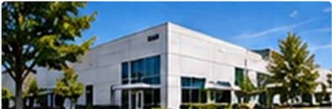
07 · Front elevation No new visible concern
